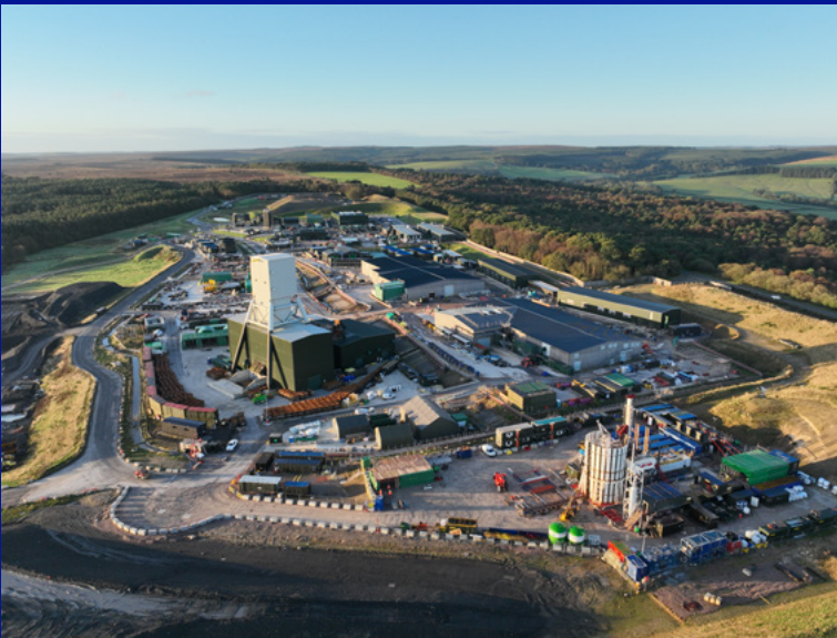
Drone view of the Woodsmith project.
