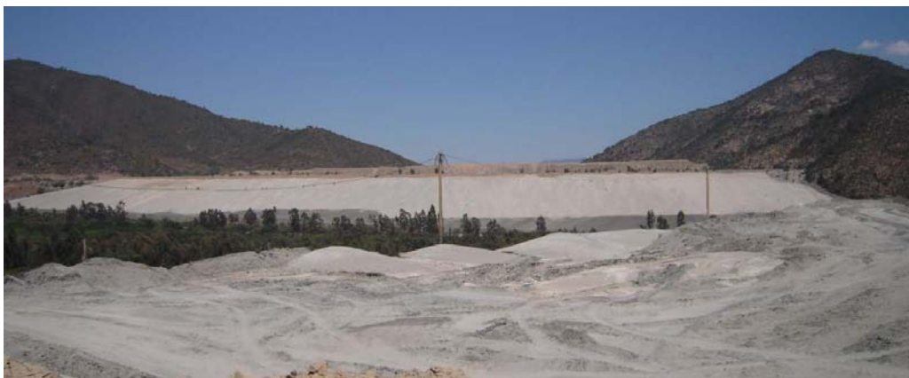
Figure 6 – View of the downstream slope of abandoned El Cobre No. 4
