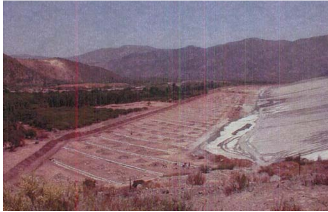
Figure 14 – View of drainage field layout
