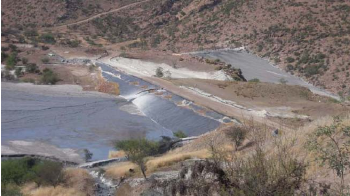
Figure 12 – View of small west impoundment embankment dam
