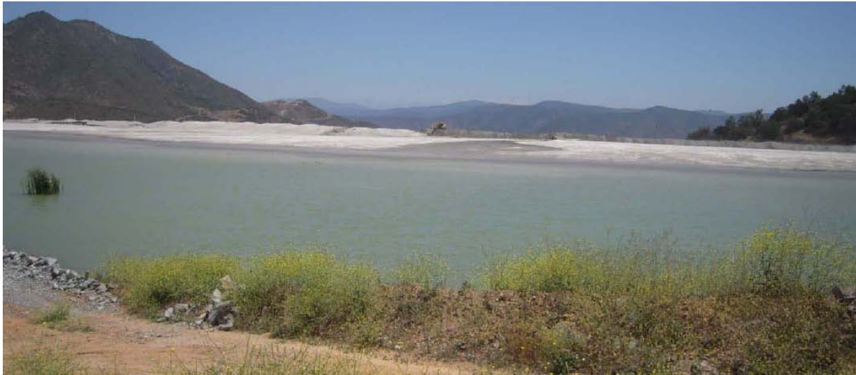
Figure 3 – Clear water pond in a slime storage area behind the impoundment embankment dam
