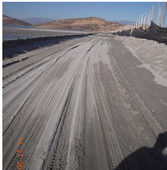
Figure 11 – View of main dam crest from east abutment, looking west
