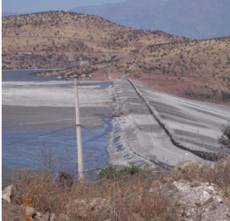
Figure 1 – Tailings slimes (left) stored behind the impoundment embankment dam (right)
