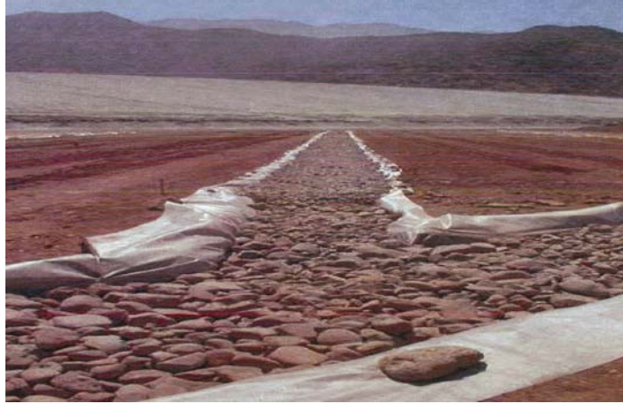
Figure 17 – View of completed drains
