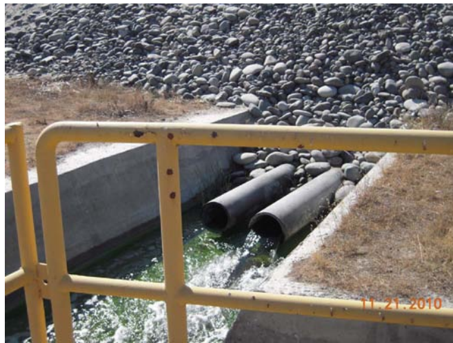
Figure 18 – View of drainage system discharge point
