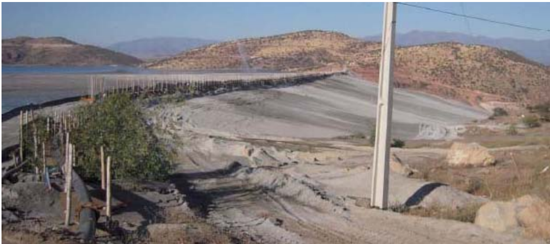
Figure 10 – View of main dam downstream slope from east abutment, looking west
