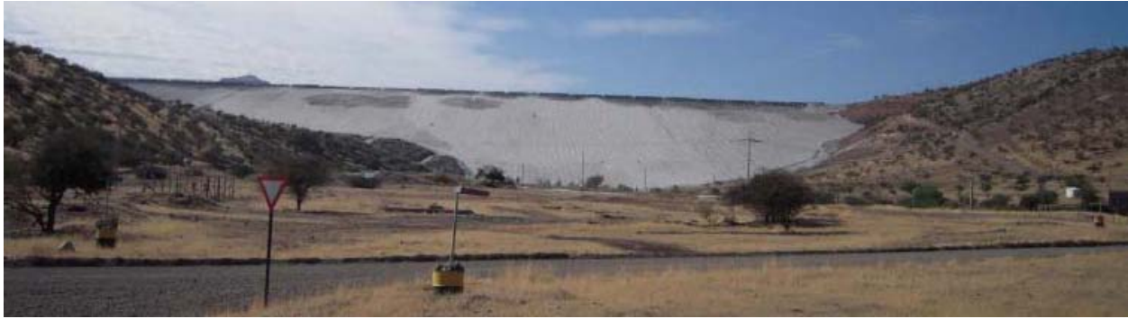
Figure 9 – View of downstream slope of main dam, looking south
